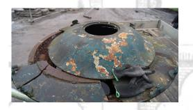
The cast domed roof had collapsed and this required repair using stitching and plating techniques. The cleaned and repaired components were then repainted using a 2-part paint system before it was re-erected on site in Alexandra Park.
