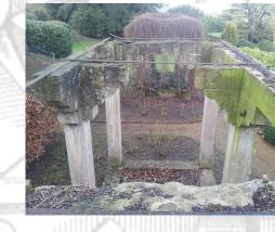
The wrought iron straps, used to stabilise the stone structure forming the pagoda, were carefully removed. These were cleaned of corrosion back to a sound metal surface and then protected with a good quality paint system. Once the stonework had been repaired, the straps were re-fitted, being re-leaded into their original locations.
