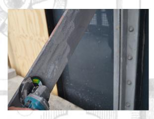
Heritage Project Contracts trialled several techniques including local blasting and using power tools with abrasive pads fitted, to strip off the loose paints leaving the ironwork ready for re-finishing with a suitable paint system.
