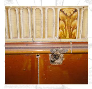
A number of specialist resins were trialled in order to identify the most suitable for repairing the damaged tiles on site. These included commercial repair systems.
