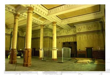
Heritage Project Contracts was appointed by Morgan Sindall to carry out trial works including the cleaning of the surviving tiles, development of a suitable repair technique for damaged tiles and to source new replica tiles to replace those that were badly damaged and missing.
